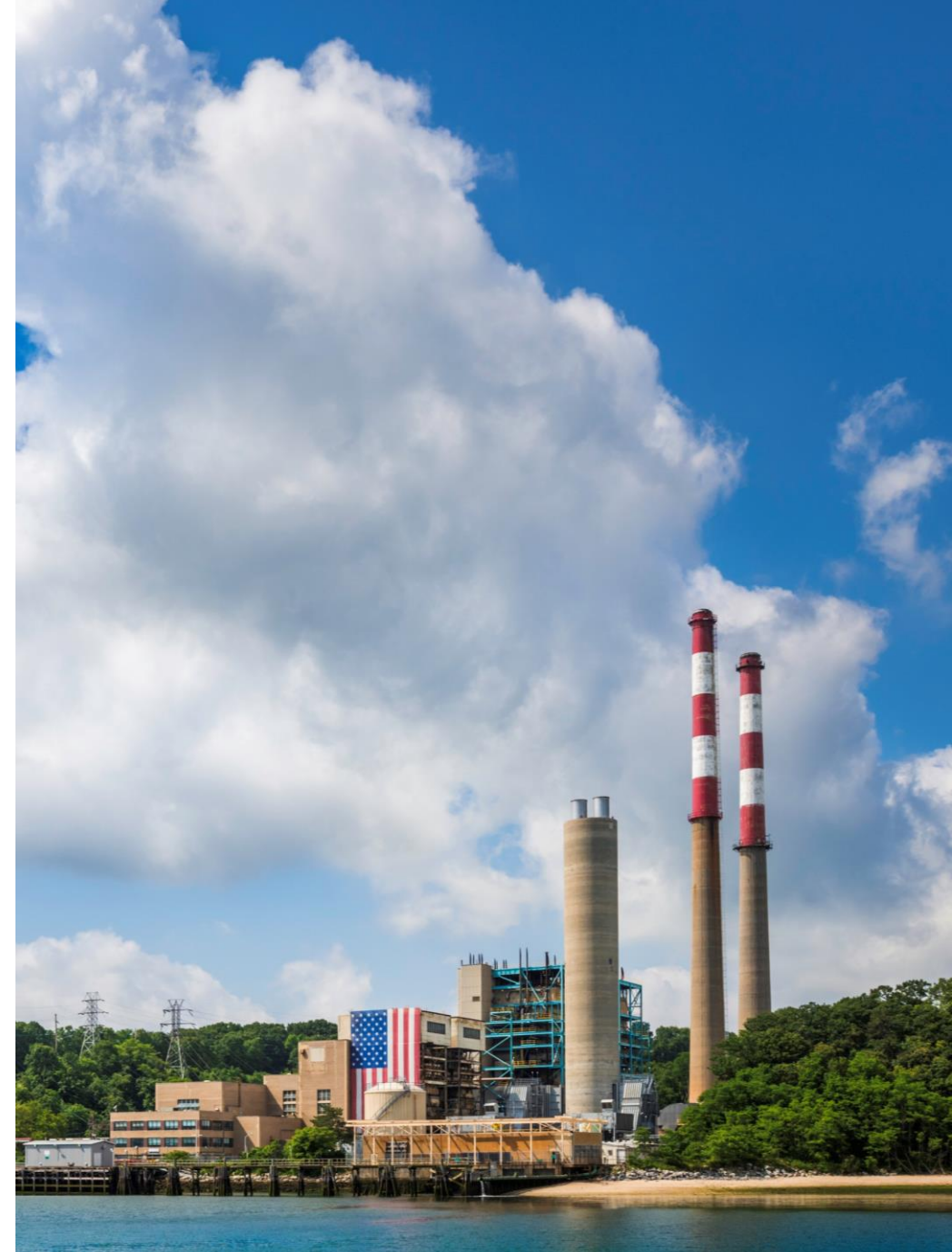
Port Jefferson Power Station
