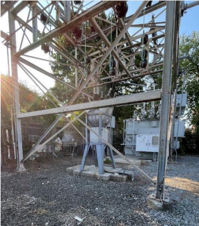
Figure 15: Roosevelt Substation showing slight rust on supporting structures, as well as a damaged ground wire
