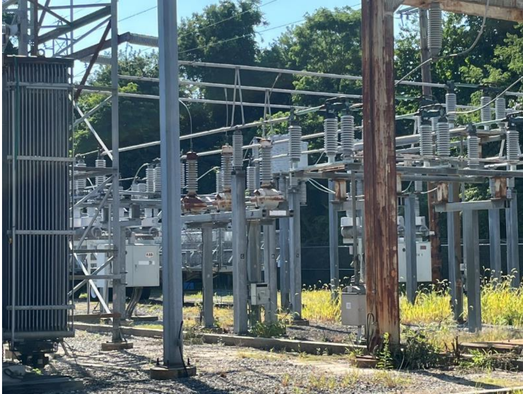
Figure 19: Peconic substation vegetation and slightly rusted support structures
