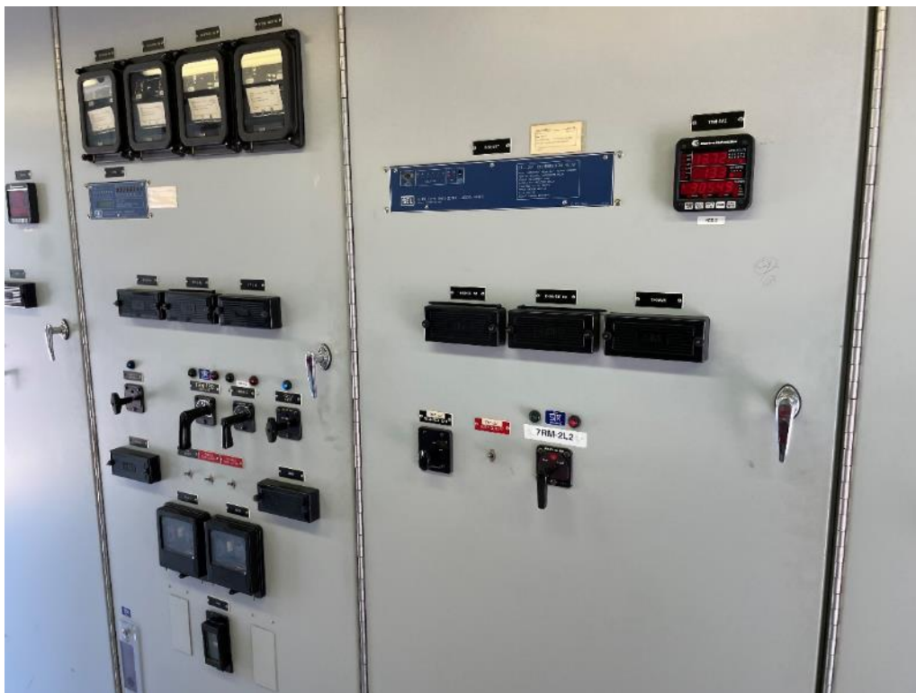
Figure 18: Bayport substations utilizes both electromechanical as well as digital relays
