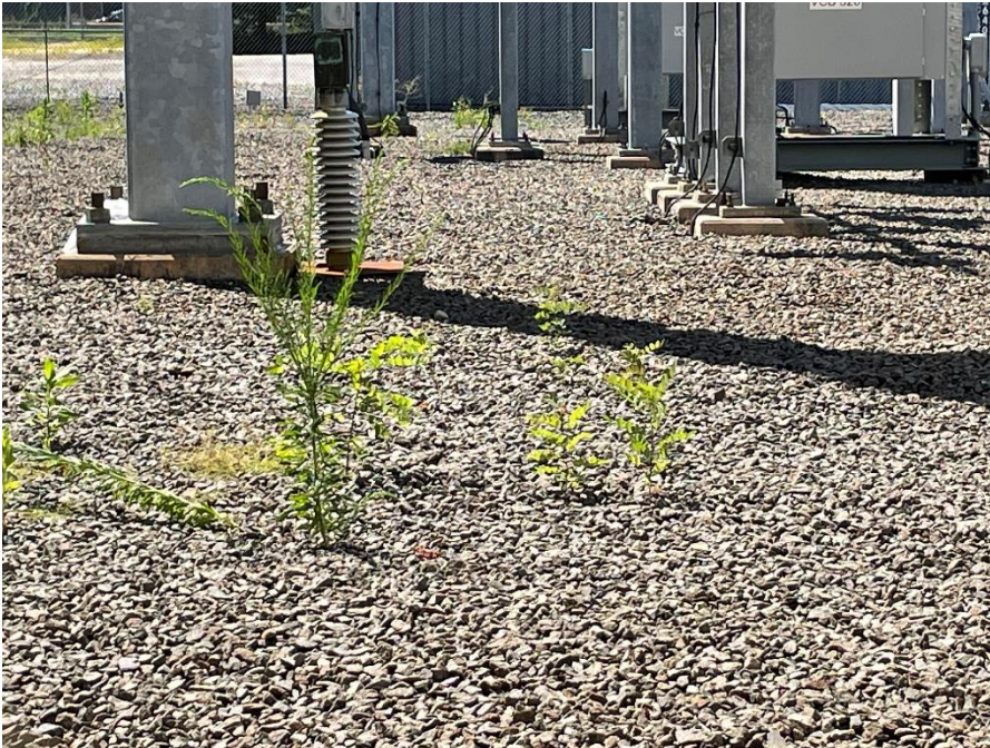
Figure 13: Ocean Avenue Substation has some weeds that should be removed.
