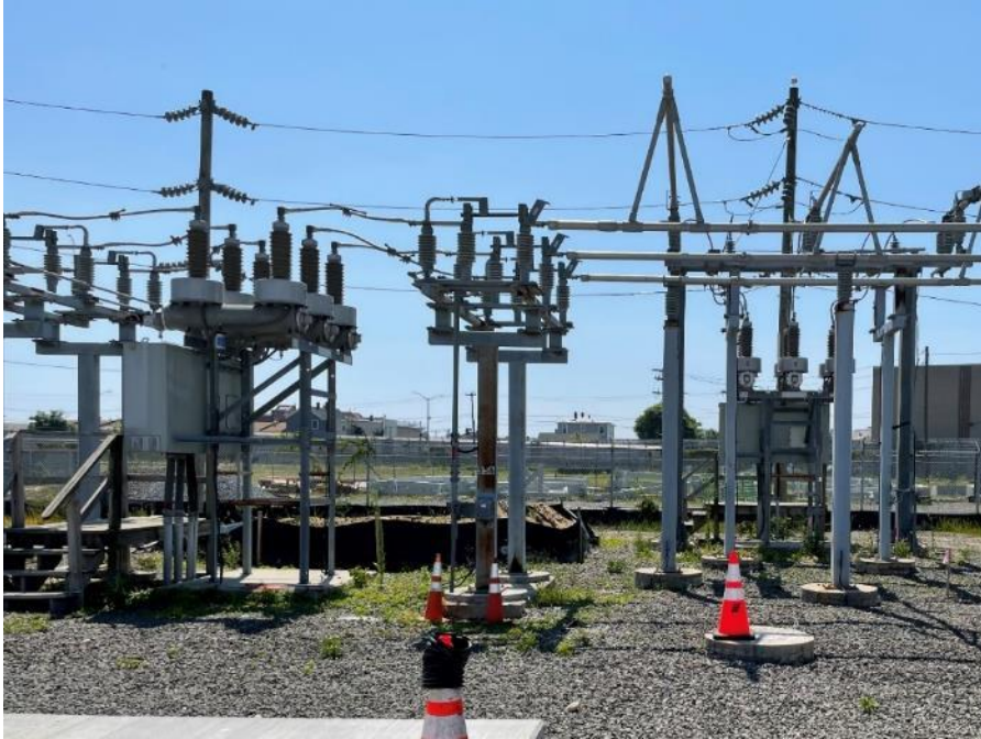
Figure 7: Rockaway Beach Substation: Rusted Transformer Cabinet and support structures
