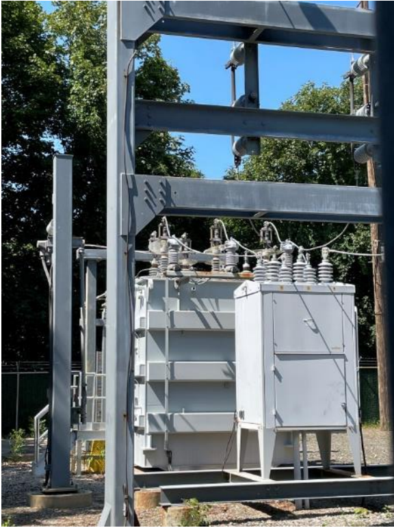
Figure 22: Orient Point substation's supporting structure showing minor amounts of rust
