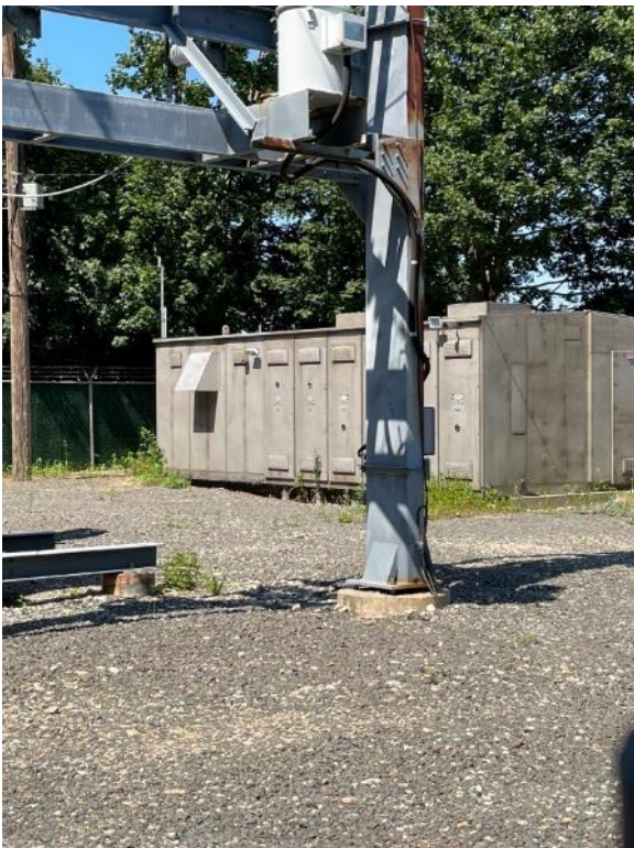
Figure 22: Orient Point substation's supporting structure showing minor amounts of rust
