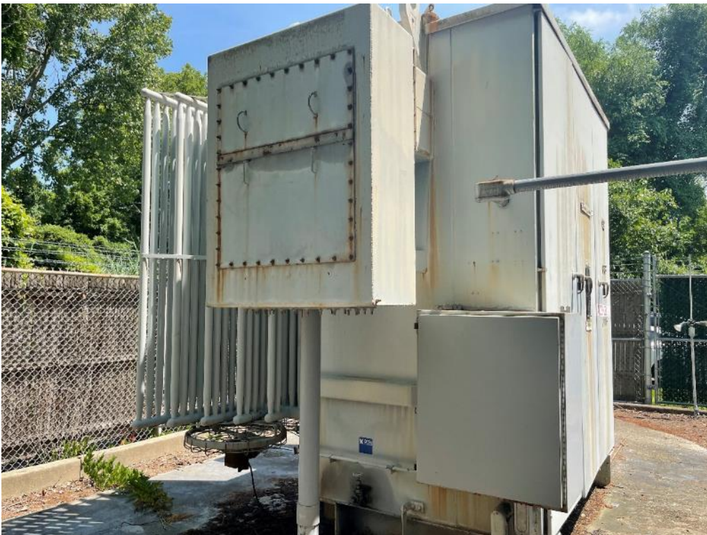
Figure 11: Kings Point Substation transformer showing minor rust and oil seepage
