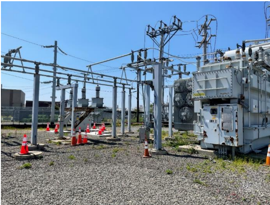
Figure 7: Rockaway Beach Substation: Rusted Transformer Cabinet and support structures
