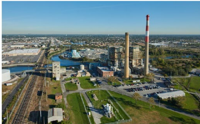
E.F. Barrett Power Station
