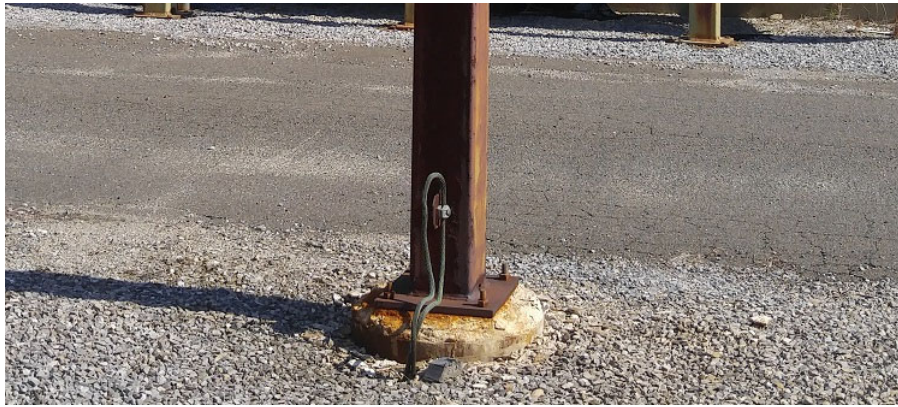
Figure 4-1: Piling Cap Deterioration
