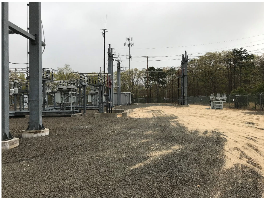
Figure 4-5: Bare Ground and Spare Equipment Transformer in Substation
