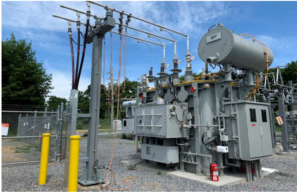
Figure 4-8: New Transformer Installation at 9Z Amagansett Substation
