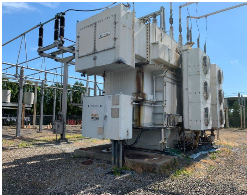
Figure 4-10: Aging Transformer in Central Islip Substation
