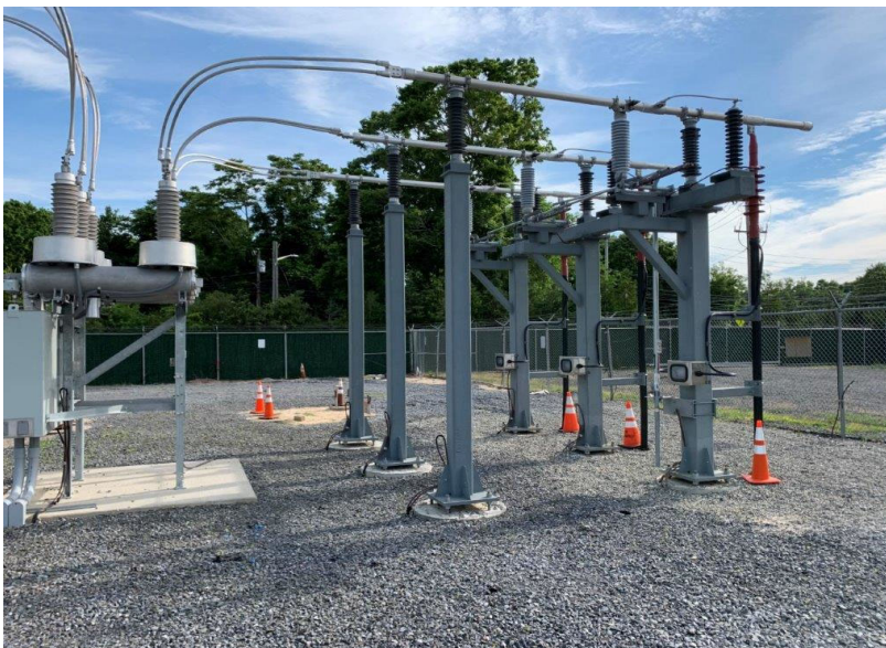
Figure 4-6: Undergrounded Circuit 620 in Eastport Substation
