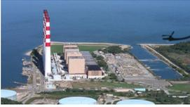
delivered by barge to the existing unloading facilities at the site and stored in two new fuel oil storage tanks of 10,000,000 gallons each. This would provide 100% capacity storage for ten days of full load oil firing on all new combustion turbine generators planned for the repowered site. The new tanks would be erected in the area of the existing #2 and #3 fuel oil tanks. The existing fuel oil tanks would be remediated and removed to make room for the new tanks.
