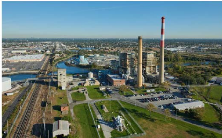
E.F. Barrett Power Station
