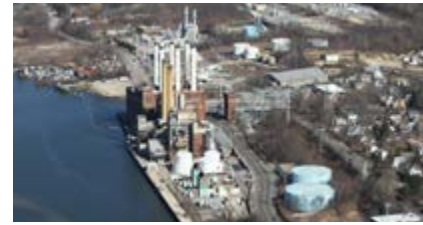
Glenwood Plant Before Decommissioning
