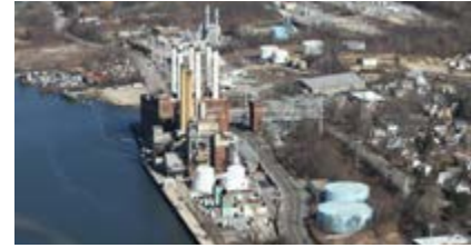
Glenwood Plant Before Decommissioning
