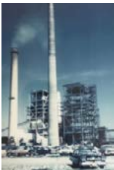
Construction of the E.F. Barrett Power Plant in Island Park, NY (1956)
