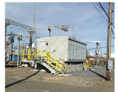
→ New Elevated Substation Raised to 500-Year Flood Level
